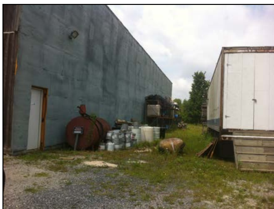
Improperly Stored Volatile Organic Chemicals - Cardinal Industries
